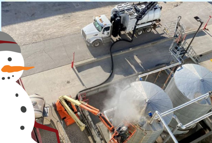
Our crew hard at work!
